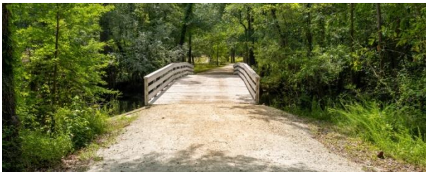
Moores Creek Bridge
