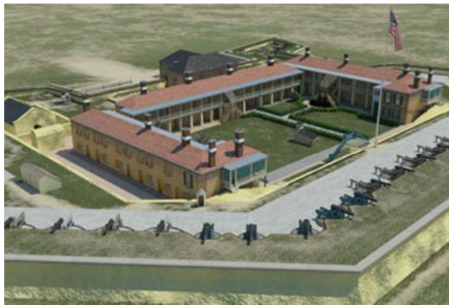
Fort Moultrie restored to Civil War era condition today
